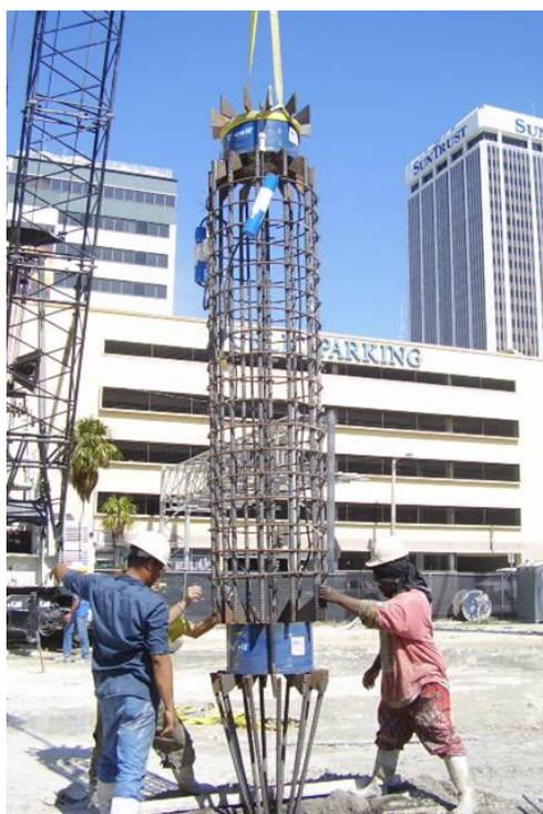
Assembly of a multi-level O-cell arrangement
