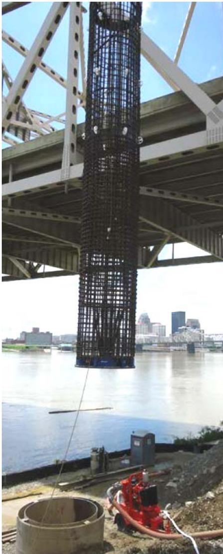
Reinforcement cage installation with O-cells
