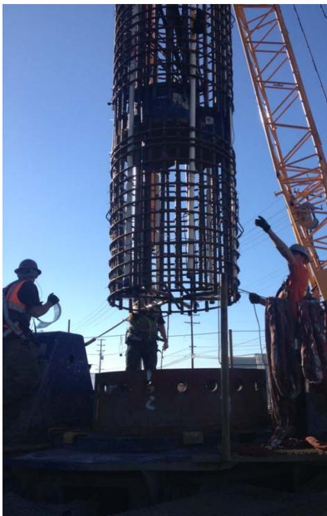
Reinforcement cage installation with O-cells
