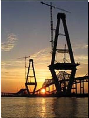
The bridge's 1,546-ft main span is supported by two 575-ft-high, diamond-shaped towers
